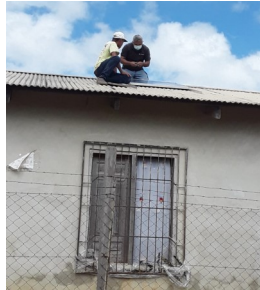
Installing solar panels
