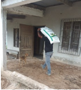
Porch ready to rebuild
